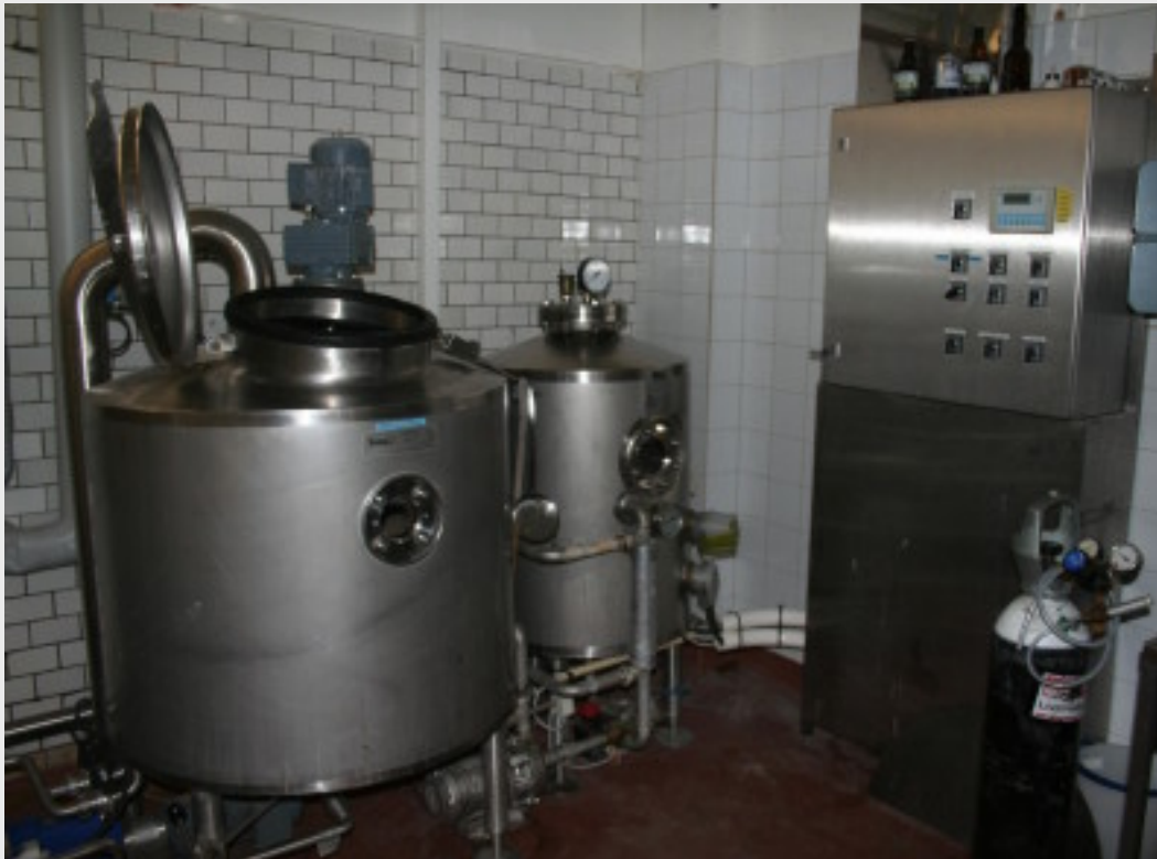
Wort Kettle, external Heating Kettle, Control Cabinet
